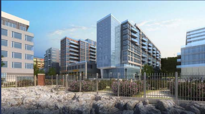
Building 8/9 at Port Imperial- Weehawken, NJ (In-Construction)
